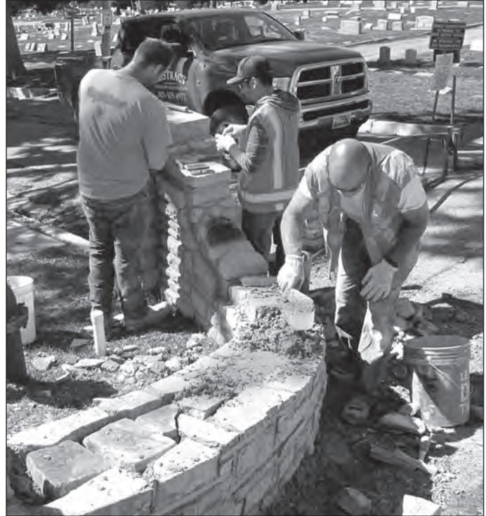
In mid-March, workers rebuild a curving cemetery entrance structure in a long-needed rehabilitation of WPA-era wall.
